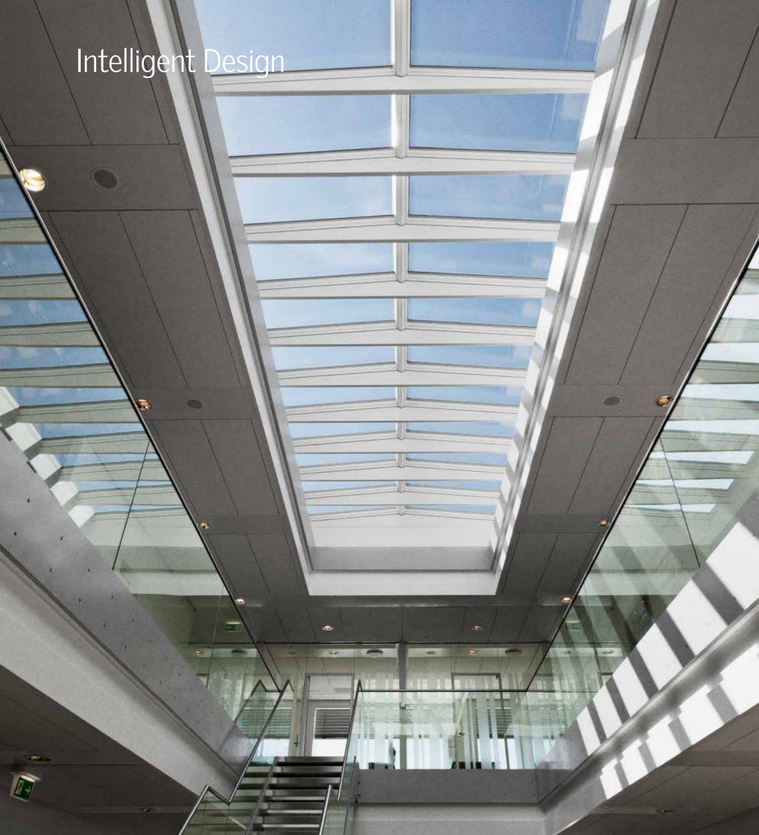
Ridgelight 5° in the ATP building, Vordingborg, Denmark – closed modules.
